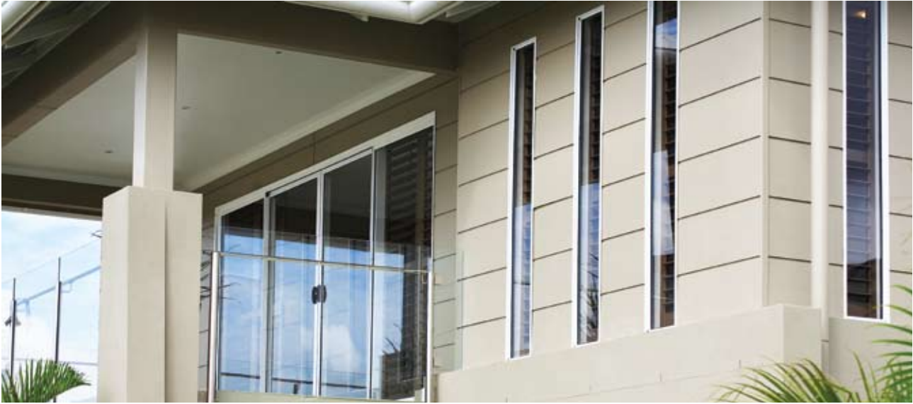
Scyon™ Stria™ cladding on Plantation Homes' Empire House at North Lakes.
