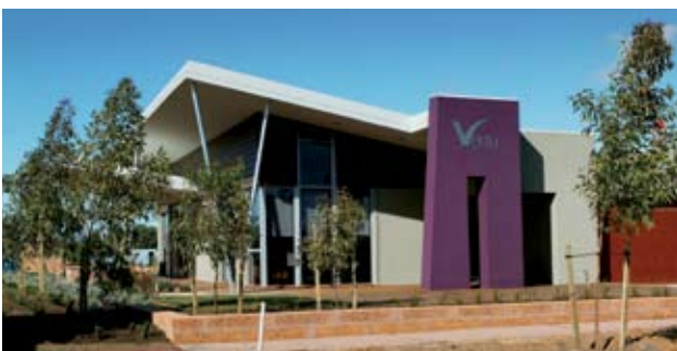
Stockland sales office. Vertu, Forrestdale, WA. Summit Homes, using Scyon™ Linea weatherboard and Scyon™ Trim, HardiTex system and Versilux lining.
