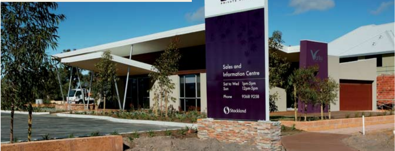
Stockland sales office, Vertu, Forrestdale, WA. Summit Homes, using Scyon™ Linea™ weatherboard and Scyon™ Trim, HardiTex® system and Versilux® lining.
