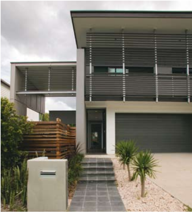
Waterline, Bulimba, Brisbane, QLD. Mirvac, using HardiFlex® sheets, HardiPanel® compressed sheets, ExoTec® facade panel and fixing system and Scyon™ Linea™ weatherboard.
