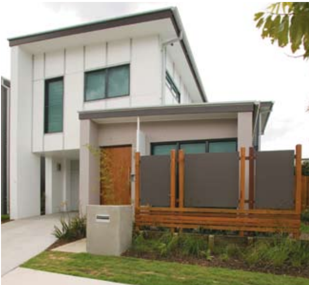
Waterline, Bulimba, Brisbane, QLD. Mirvac, using HardiFlex sheets, HardiPanel compressed sheets, ExoTec facade panel and fixing system and Scyon™ Linea weatherboard.
