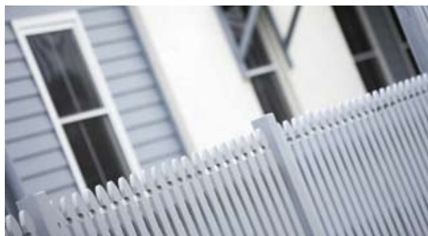
Tullimbar Village, NSW. Miltonbrook, using Scyon™ Linea™ weatherboard.
