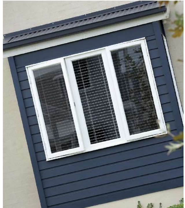
Tullimbar Village, NSW. Miltonbrook, using PrimeLine Newport weatherboard.
