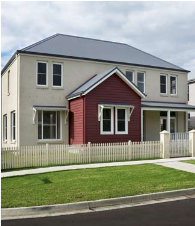
Tullimbar Village, NSW. Miltonbrook, using PrimeLine® Newport weatherboard.
