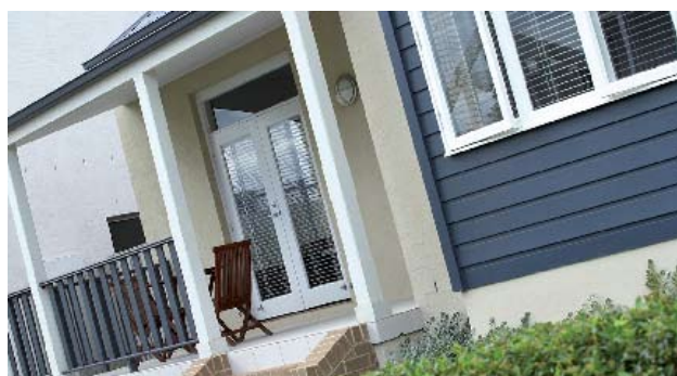
Tullimbar Village, NSW. Miltonbrook, using PrimeLine Newport weatherboard.
