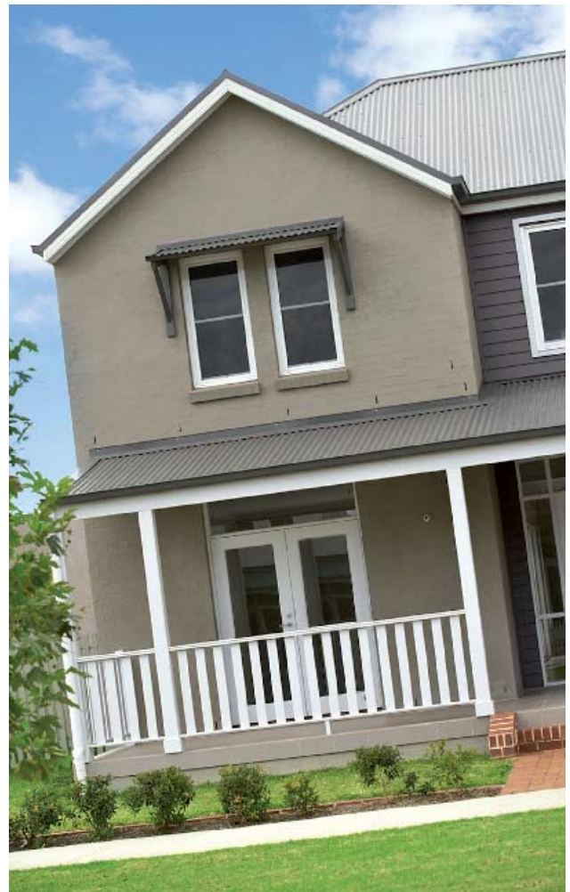
Tullimbar Village, NSW. Miltonbrook, using Scyon™ Linea weatherboard.
