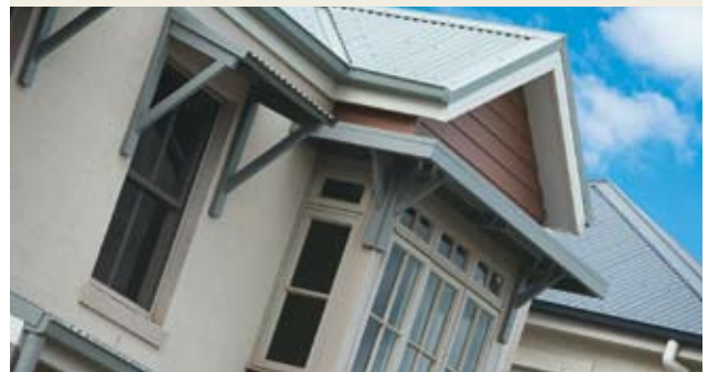
Tullimbar Village, NSW. Miltonbrook, using Scyon™ Linea weatherboard.
